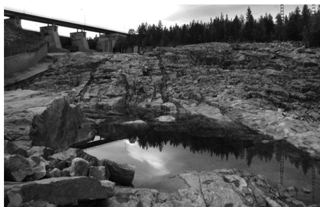
Figure 2. The spillway channel in Ligga.
