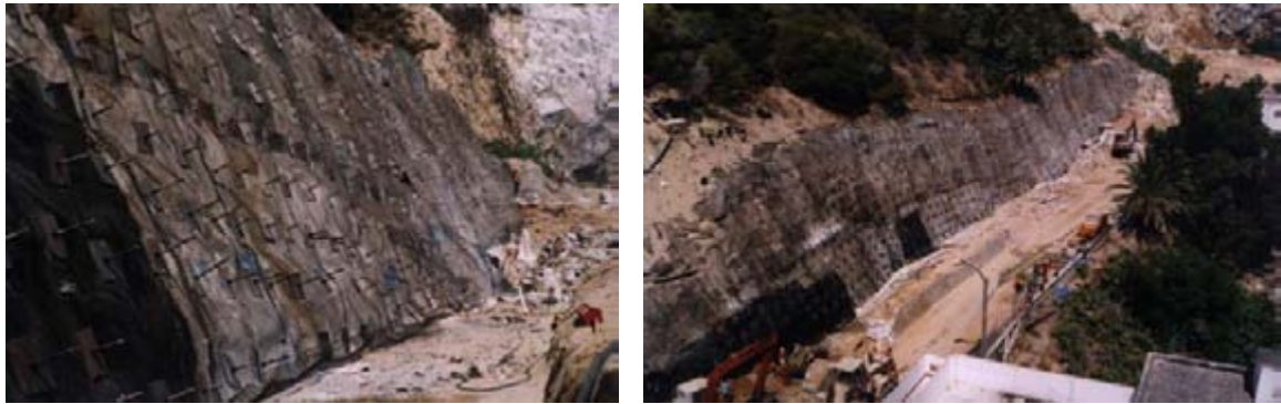
Fig. 13 a 14: Soil Nailing at Sir Herbert Miles Road, Gibraltar
