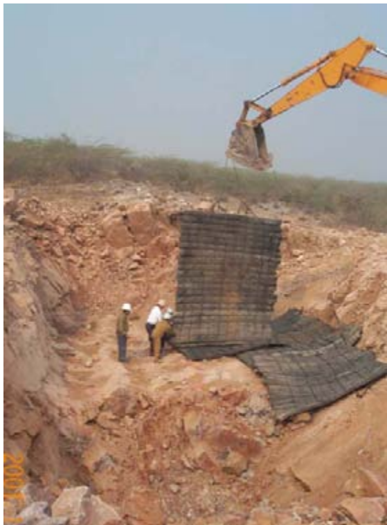
Figure 3 Blasting mats are being put on top of the bench at the test blast Mattor appliceras ovanpå pallen vid provsprängningen
