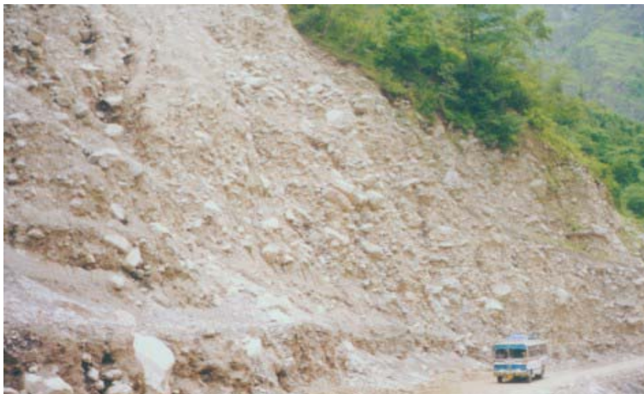
Fig. 1: Lambagarh Slide Chamoli District, Uttar Pradesh, India
