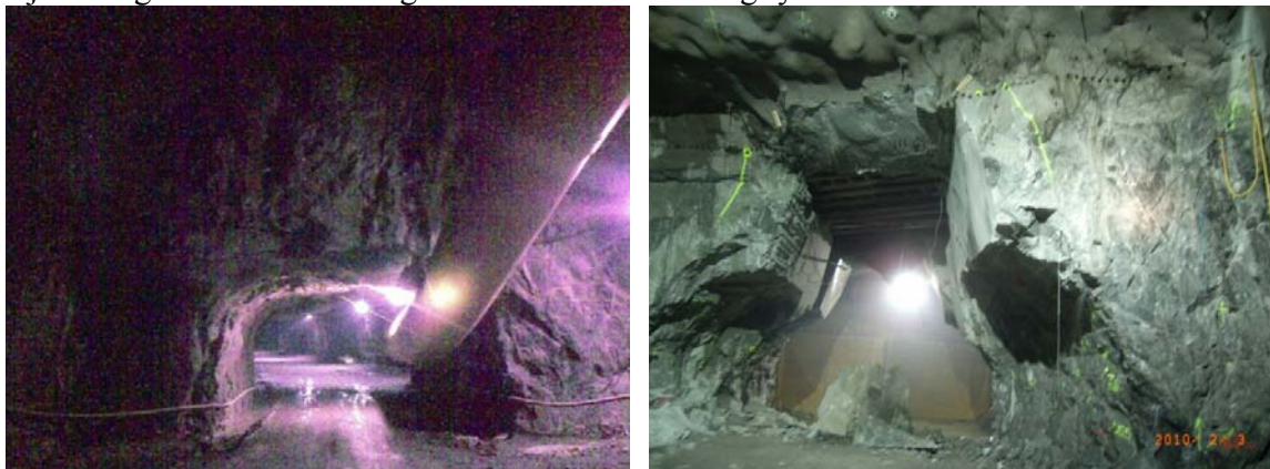
Figur 7. Korsning mellan Tunnelbanan och Tunnel 313 Intersection between the Metro and the Tunnel 313.
