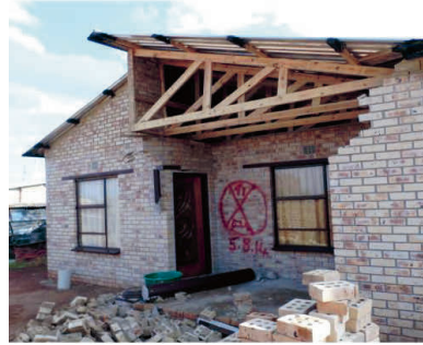
Figure 1: Damage to dwellings in Khuma as a result of the M5.5 earthquake on 5 August 2014 (photographs Prof. Herbert Uzoegbo, University of the Witwatersrand)
