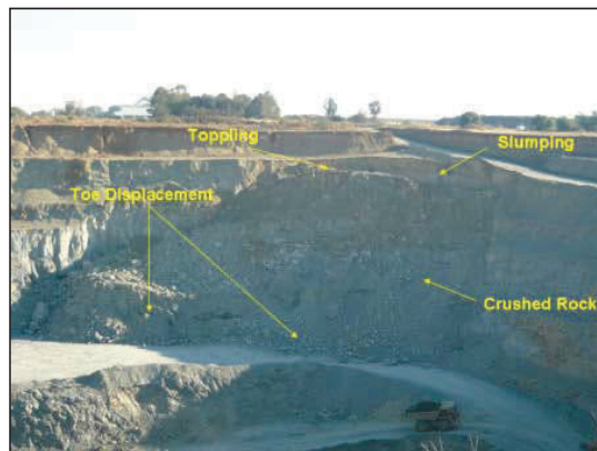
Figure 4: Photograph of the First Stack-Scale Failure in the VO Unit
