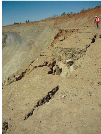
Figure 5: Failure in VO - September 2010
