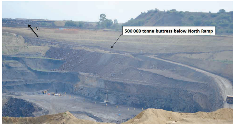
Figure 15: Buttress below the North Ramp. Photo taken in December 2012.
