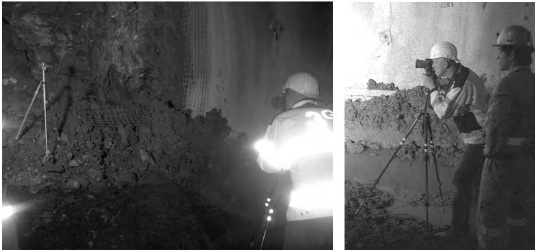
Figure 12. Data collection using ShapeMetriX3D during face documentation. The camera is mounted on a tripod. A range pole at the face provides scale and vertical reference.
