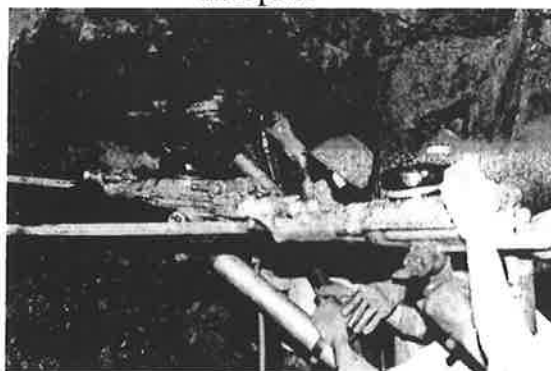
Drivning med handhållna borrar. Excavation with hand held drills.
