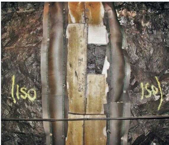
Figure 3.11 Patched and repaired drain in the Bergträsk tunnel (Photo: Erik Stål, 2011).
