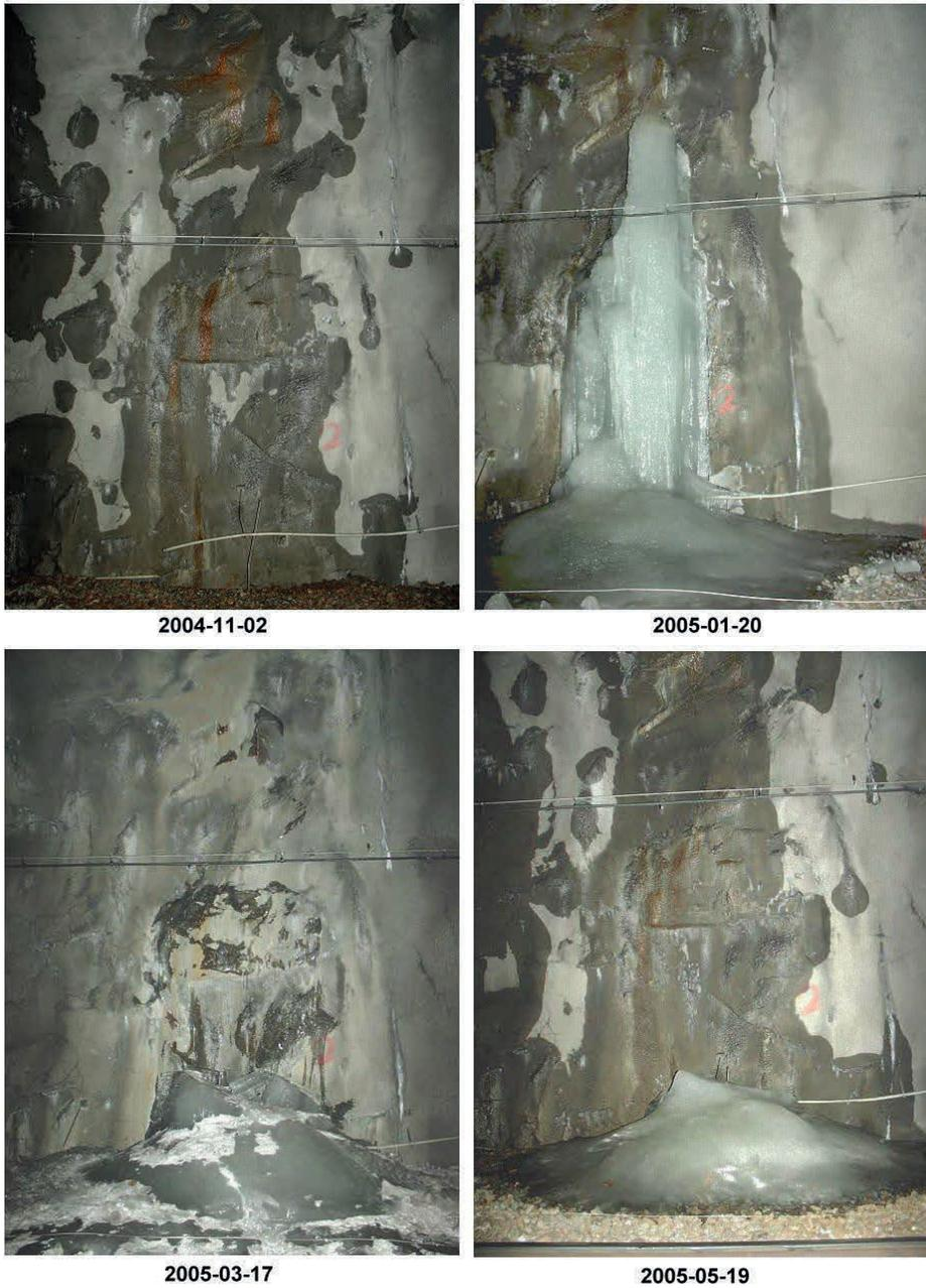
Figure 3.4 Differences between the four inspections in the Glödborget tunnel at chainage km 816+345, 185 m from the south entrance (Andrén, 2008).
