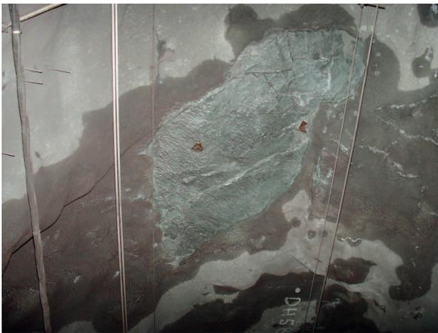
Figure 1.3. Shotcrete fall-out from 2003 in the roof of the Nuolja tunnel (Andrén, 2008).
