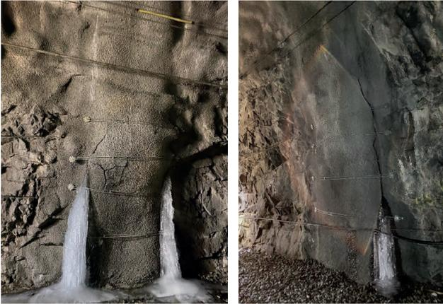
Figure 3.12 Cracked shotcrete over drain mat in the Bergträsk tunnel (Photo: Stabilt, 2020).
