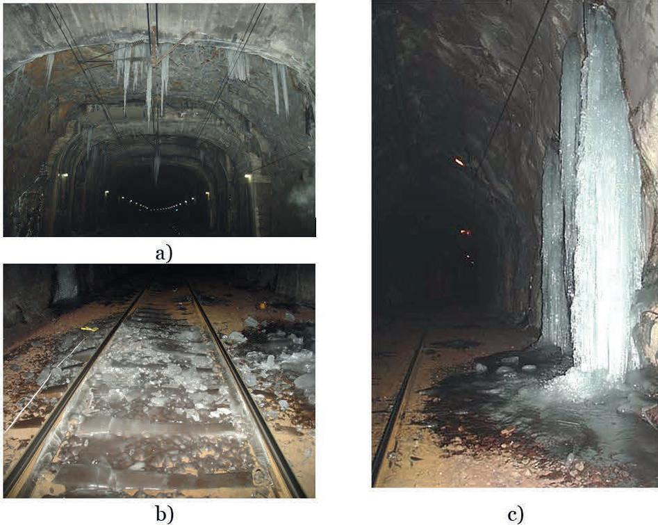
Figure 3.2 Typical problems with ice formations that might develop in unlined tunnels (Andrén, 2008):
