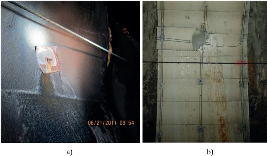
Figure 3.9 a) Leakage around rusty bolt and bolt washer, Skogsby tunnel (Tyréns, 2011).
