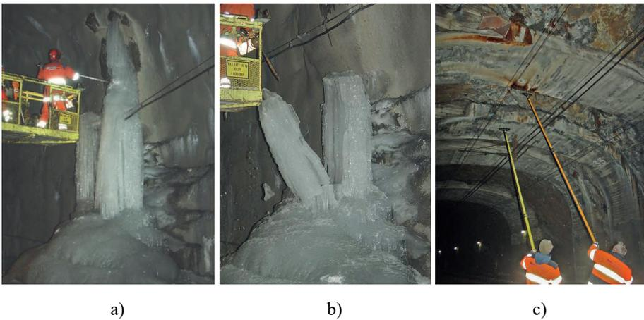
Figure 1.2 a) and b) Removal of ice pillar in the Glödsberget tunnel (Andrén, 2008).
