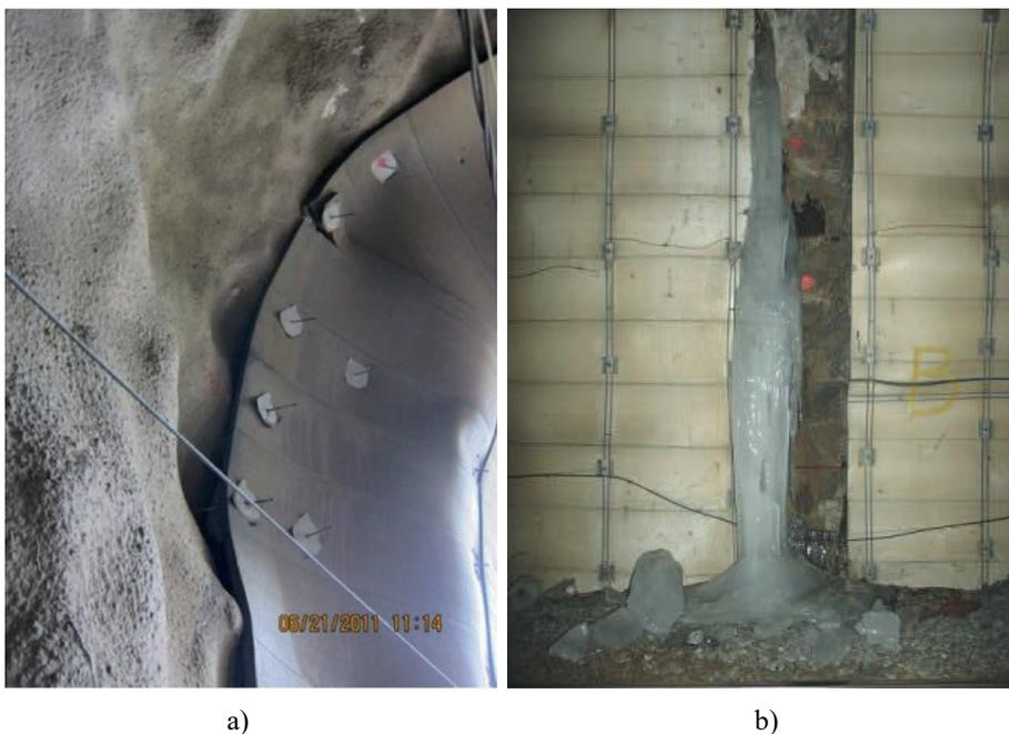
Figure 3.8 a) Drain mat not sealed against the tunnel contour, Margreteberg (Tyréns, 2011).
