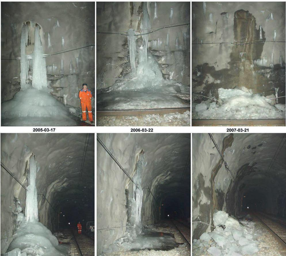
Figure 3.5 Comparison at chainage km 816+665 (505 m from the south entrance) in the Glödborget tunnel in March 2005, 2006 and 2007 (Andrén, 2008).
