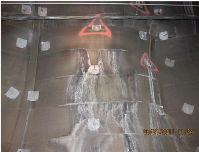
Figure 3.10 Leaking welded splices, Margreteberg (Tyréns, 2011).
