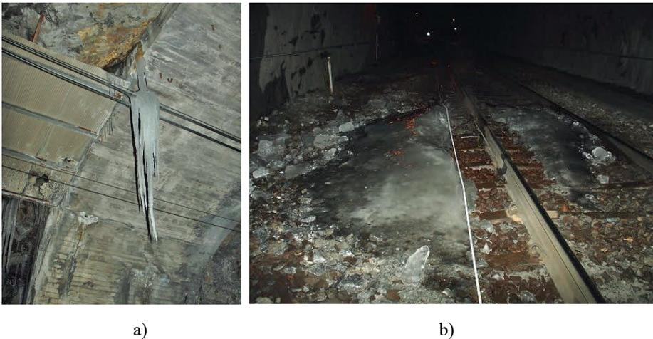
Figure 3.14 a) Icicle in the roof of the Rönninge tunnel (Andrén, 2008).
