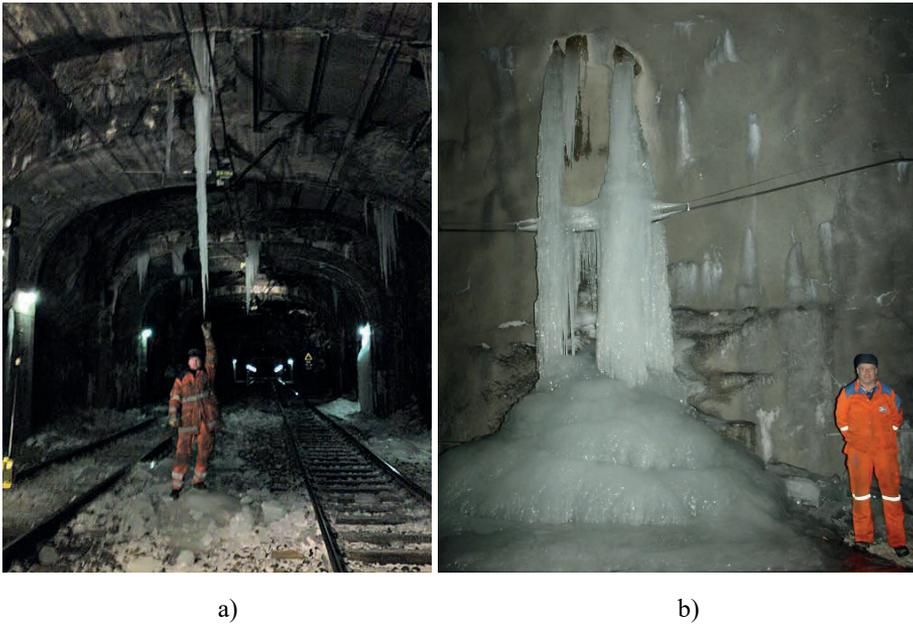
Figure 1.1 a) Icicle in the Rönninge tunnel (Photo: Infranord, 2010).
