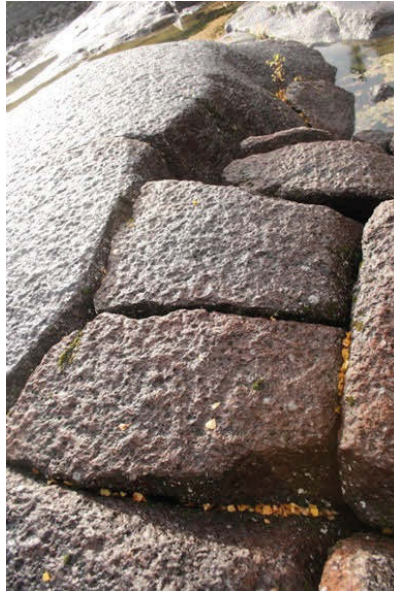
Figure 35. Large apertures are observed.
