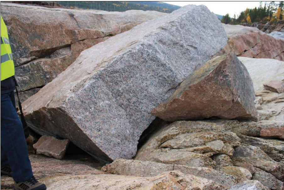
Figure 16. Large block formed by the dominant sub-horizontal structures intersected by the two random vertical joint sets, which has been dislodged by water pressure.
