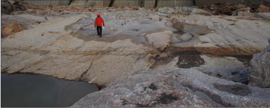
Figure 19. Peeling of the rock surface above the plunge pool by water jet. The surface has been engineered for controlled erosion.
