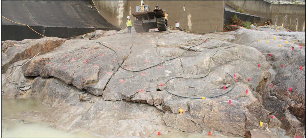
Figure 31. Shallow dipping joints that form flat lying slabs near the hydraulic jump slope.
