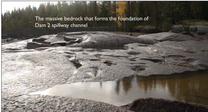
Figure 28. Massive granitic bedrock at Dam 2 spillway channel.
