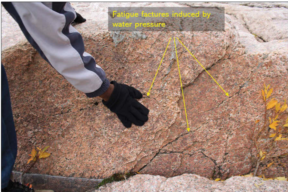
Figure 18. Fatigue fractures induced by water pressure.
