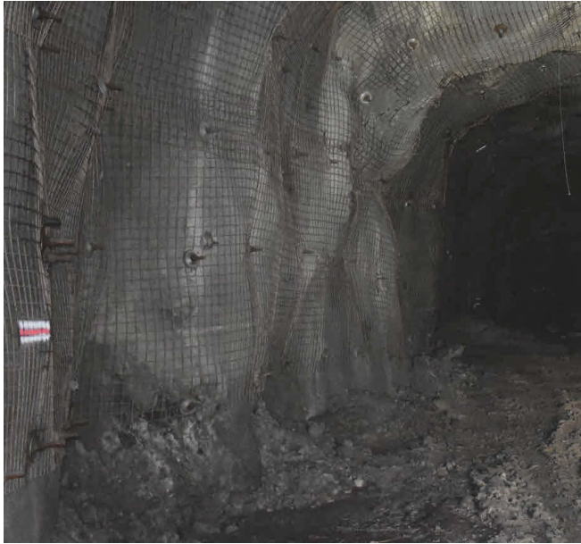
Figure 37: White-red-white reference lines marked on opposite walls for level-line projection.
