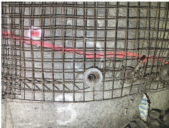
Figure 33: Convergence monitoring point in PR996 crosscut 4090, S3.
