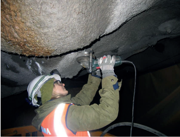
Figure 2-3. Grinding of the bolt end.
