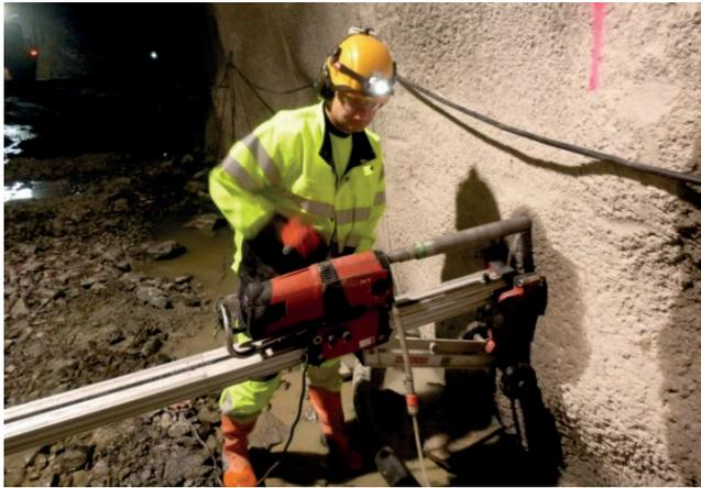
Figure 2.2 Collection of core samples with Hilti DD200 diamond core drill.
