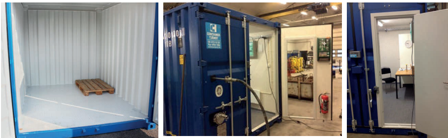
Figure 7. Photos of container before (left) and after rebuild to mobile test laboratory.
