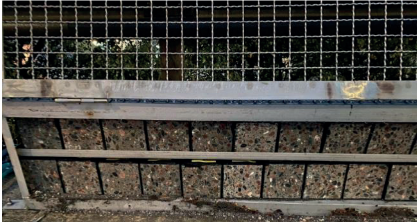
FIGURE A6.4. October 2020 permanent marker numbering had been removed from power washing and weather.
