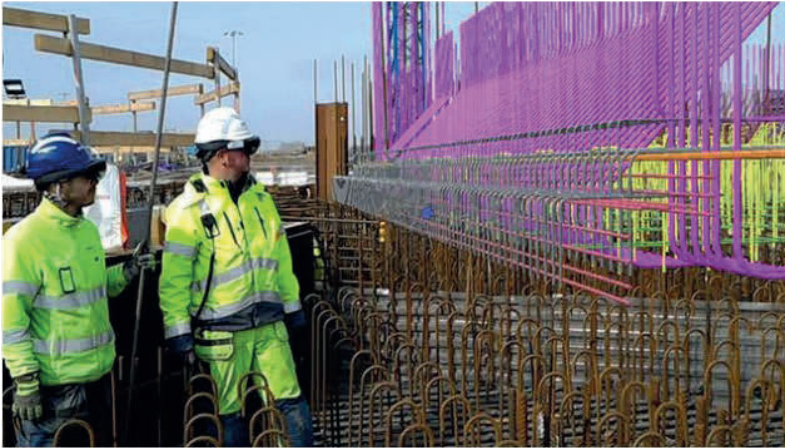
Figure 14. Building site through the HoloLens glasses (Nohrstedt, 2017).
