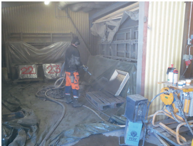
Figure 2.2. Spraying of a test box with shotcrete.
