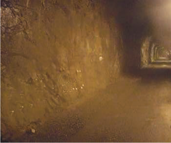
Figur 2 Åspötunneln (The Åspö tunnel)
