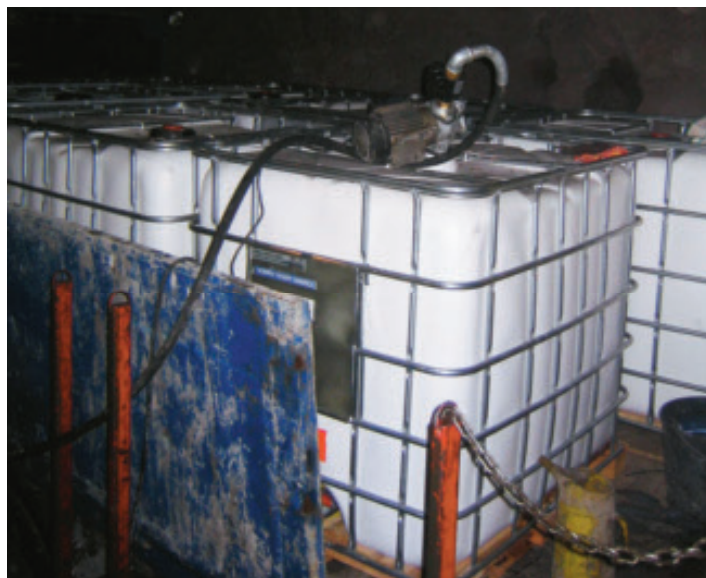
Figure 3-2. 1m 3 container with silica sol and a saline solution from a project in one of the Telia tunnels.
