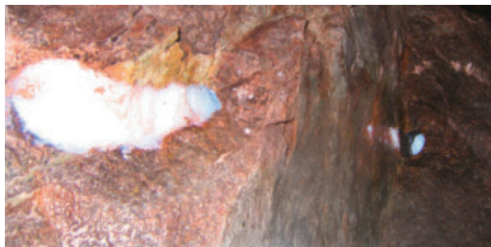
Figure 3-8. A good silica sol plug in a borehole. Image from Hallandsås.
